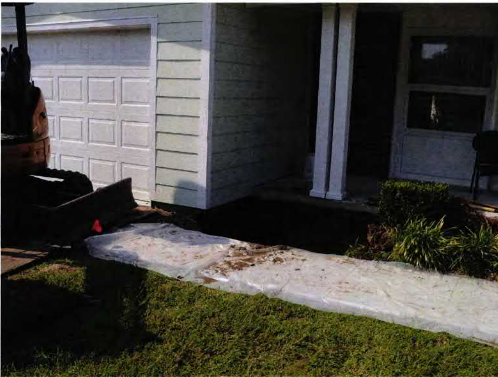
Picture 2: UST 200Balsam excavation in progress.
